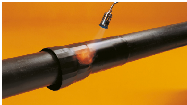
Heating the BXSJoint. Second seal
